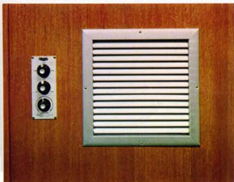
Optional air conditioning has reverse cycle for cooling or heating.
