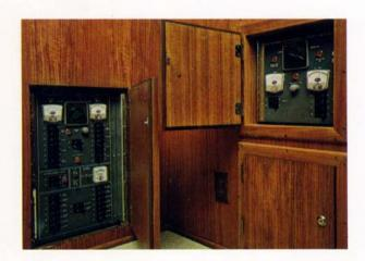
An example of engineering excellence is the comprehensive and complete electrical system. The master electric control panel is installed in convenient location for easy visibility and access. It provides central control and protection for both 12 volt and 110 volt systems. Electric control panel with circuit breakers, distribution switches, voltmeter, ampere consuming meter, battery condition meter, indicator light, polarity check and navigation lights.
